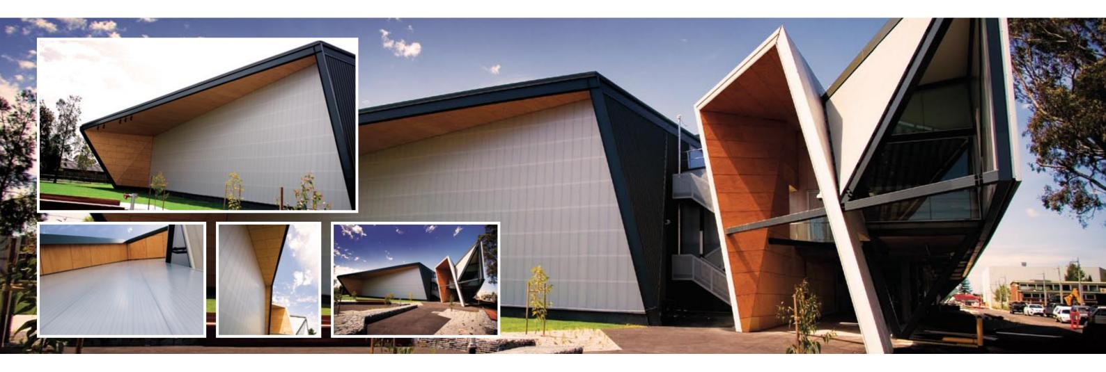
Nanokote was engaged to apply its EcoBarrier<sup>TM</sup> anti-graffiti coating to the Danpalon polycarbonate walls for the Victoria University Sunshine Construction Futures project. The Danpalon substrate was particularly susceptible to permanent damage from both graffiti markers and removal agents that would result in permanent damage to the surface.
