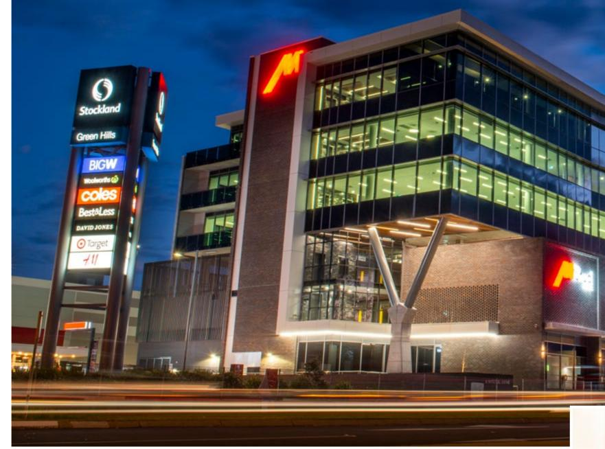
bespoke onsite fabrication jigs in order to position and fabricate the item. It was craned into place at night requiring a full road closure of the busy main street.
