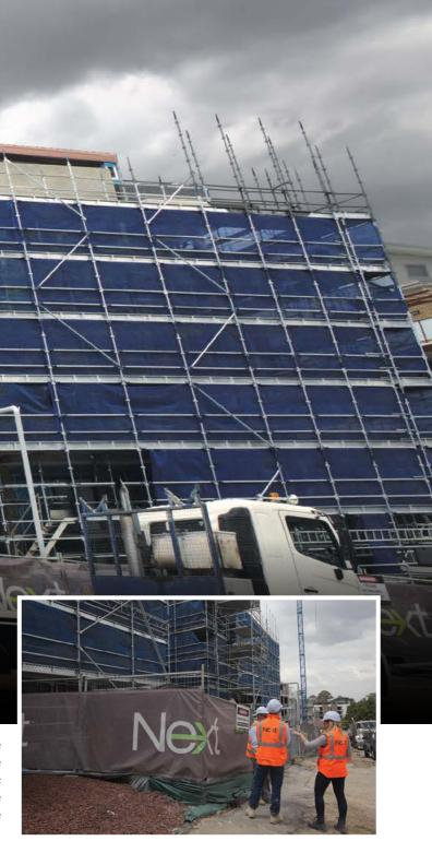
wall solution was decided to be the best alternative to the usual, Hebel wall system. The speed panels unique tongue and groove system with top and bottom racks translated to a quick installation, and they also boast excellence fire and acoustic properties. Another life-saving option was the Trafalgar Fyrebox system, which has ensured the residential complex is fire compliant and equipped in the event of fire emergency to ensure all services are stopped – a simple and effective solution.
