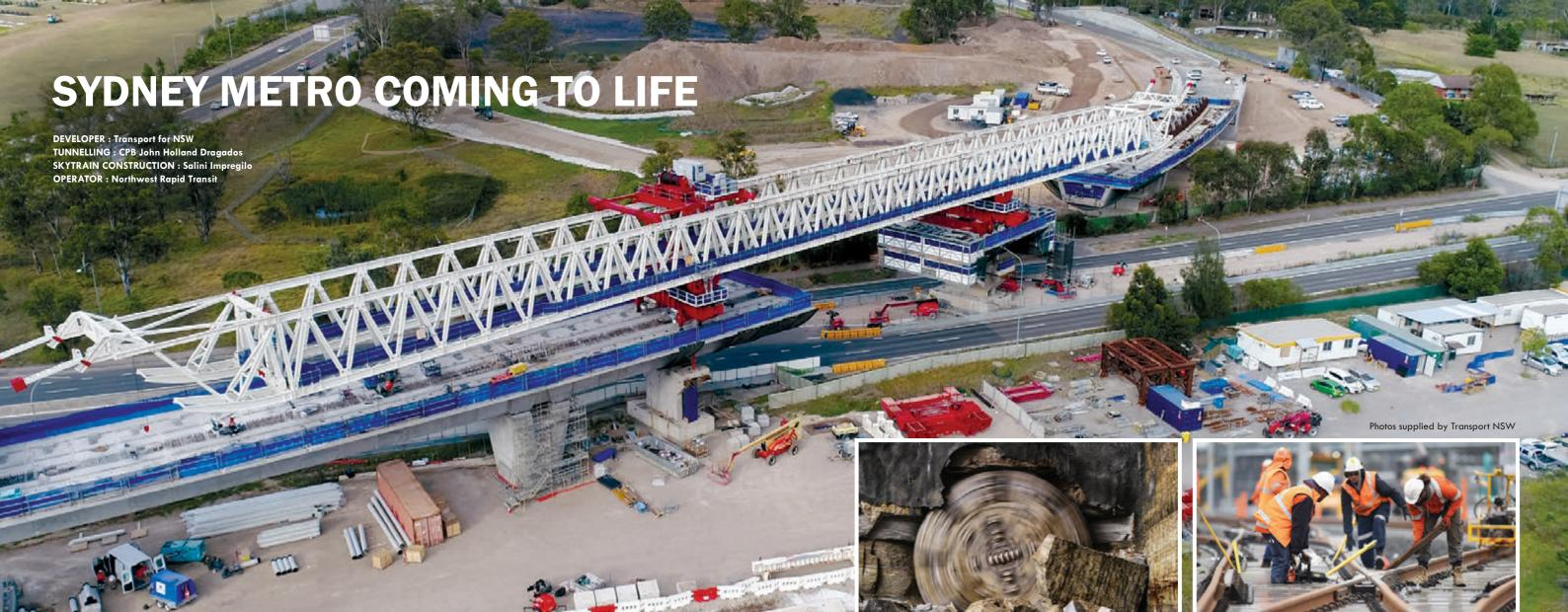
The \$8.3 billion Sydney Metro Northwest is Stage 1 of Sydney Metro. It includes the skytrain - a 4km elevated viaduct including the first cable-stayed rail bridge built on a curve in Australia.
