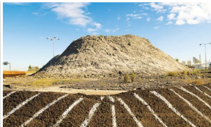
BHP Mayfield Closure Area Stage 1- The identification and management of Spoil from 1050m of two open drains treating 9038m3 of PASSnsite
