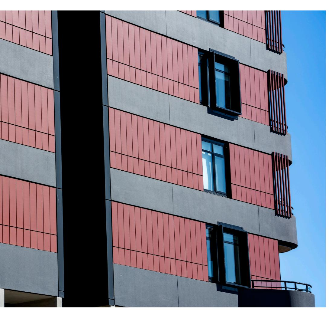
Australian Cladding Specialists (ACS) were appointed under a design and build contract to supply and install external façades to Stage 1, including terracotta and aluminium cladding to all three towers in the complex.
