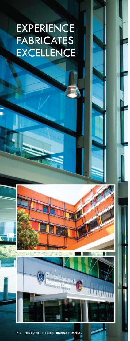
o steel project is too large or complicated for Toth Engineering, and Robina Hospital's structural steel work is proof. Toth Engineering designed, fabricated and installed steel work included columns, bridges, roof structures, walkways, sunshades, and facade structural steel including mullions and window heads. All in all, 450 tonnes of certified quality workmanship was supplied and installed over 18 months from shop drawing to final erection.
