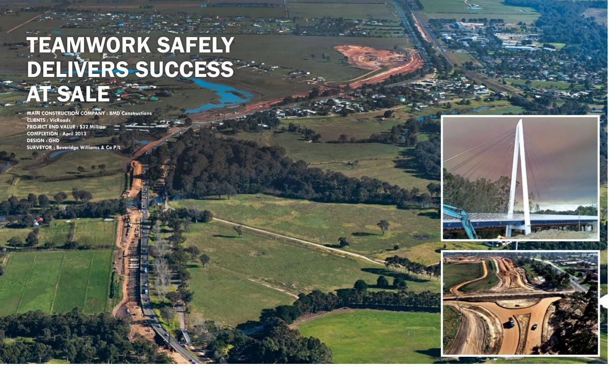
BMD's Princes Highway East Duplication – Wurruk to Sale section comprises 4.5km of dual carriageway, four new road bridges, 6 refurbished road bridges and an architecturally-designed 90 metre cable stay pedestrian bridge.
