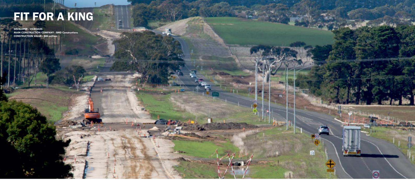
The Princes Highway Duplication project involved widening and upgrading 23 kilometres of highway to a four-lane divided road that will improve safety, travel times and reliability between Waurn Ponds to Winchelsea. It also included the construction of a new bridge over the Warrnambool-Geelong railway line at Buckley.
