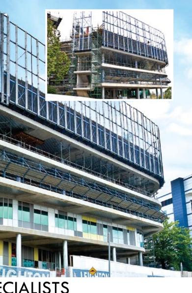
"However, our specialised team of engineers were able to overcome this issue through the design and development of specific formwork systems that are designed to withstand the sheer pressure and weight of this structure," he said.
