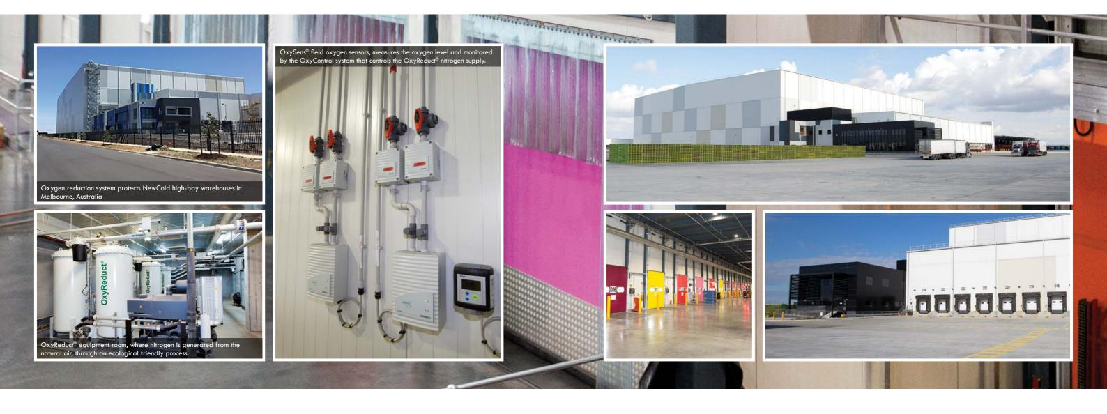
At the NewCold Advanced Cold Logistics Facilities, a fire prevention solution is installed that uses an oxygen reduction system to prevent damage from both fire and sprinkler water, as well as ensuring time sensitive logistical processes are protected. The solution comes from WAGNER Group GmbH based in Langenhagen Germany, realised with its local subsidiary WAGNER Fire Safety Pty Ltd.
