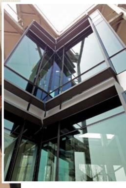
The façade is predominantly comprised of Unitised Curtain wall with double glazed units, the majority with a jockey sash for acoustic purpose, and fire rated A2 aluminium cladding. The façade also includes window walls at lower levels, a skylight and glazed cloister.
