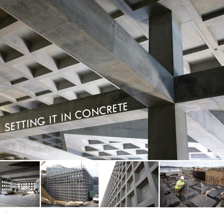
22,000m<sup>2</sup> of in-situ concrete slabs were put in over three internal floor levels and two roof levels. Total approximate tonnage of reinforced steel was in excess of 800 tonne with over 8500m<sup>2</sup> of reinforcing mesh. Stephen Little Constructions supplied 1940m<sup>2</sup> of plain precast panels and1400m<sup>2</sup> of waffle pod precast panels with 332m<sup>2</sup> precast floor beams.
