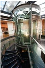
A t MONA, even the lifts are ultra-modern works of art, custom x 4200 long x 3500 high, enabling shifting of some of the Museum's designed and built by Independent Lifting Services Pty Ltd (ILS). extremely large artworks. The lift is powered by 2 roped hydraulic
