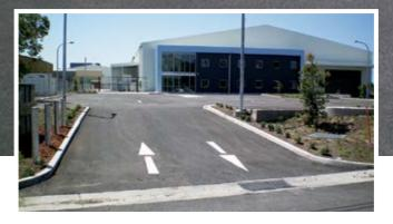
The Midal Cable facility offered almost every kind of engineering challenge - exactly the kind of project Bolte Civil thrives on. The company's scope included all the civil works, from geotechnical investigations and testing, survey setout and early enabling works through to bulk earthworks and detail excavations in watercharged ground, pavement works, stormwater drainage, detention tank construction, retaining walls, carparks, asphalting, kerbing, and erosion and sediment works.
