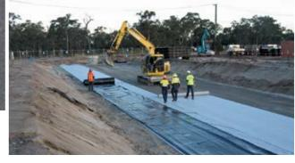
Formworker/Pit Builders, Plant operators, Pipelayers, and Civil Labourers. Plant owned by Bolte Civil used on the project included excavators, Positrack (Multi-Terrain Rubber Tracked loader), 12ton Padfoot Rollers, 12ton Smooth Drum Rollers, Grader, Watercarts, Cat 953 Traxcavator, plus Arrow Kerb & Gutter Extrusion Machine.
