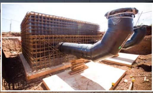
Over a period of 18 months, Pipecon installed 30km of 800mm diameter GRP for the Melbourne to Geelong Pipeline, stretching from Tarneit to Little River. It was not an easy task, with the challenges including two open cut river crossings, demanding timeframes and high quality expectations.
