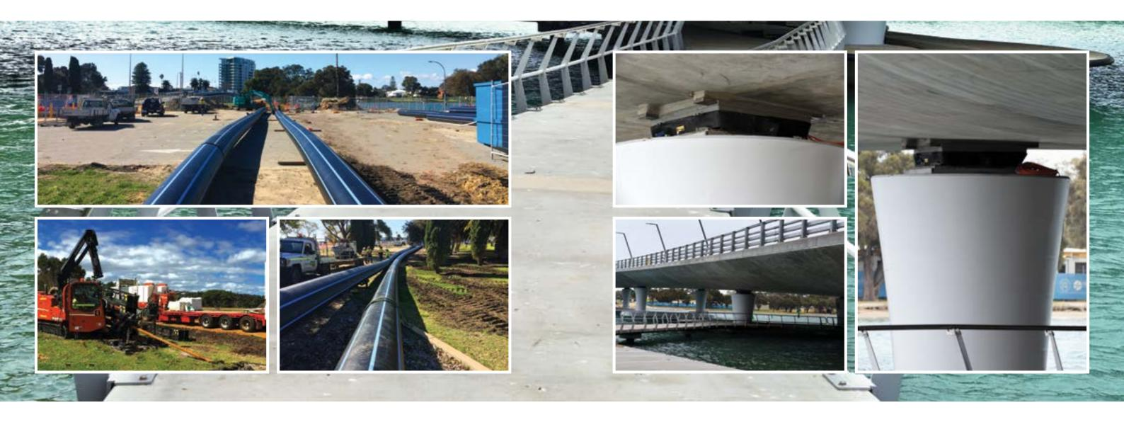
Specialists in directional and vertical drilling, Power On Cabling were chosen to lay the gas and water pipes for the Mandurah Traffic Bridge Replacement project. Unlike the old bridge, the utility pipes do not run alongside the structure, instead they sit deep within the river bed. Power On Cabling were the only company in the state with the right expertise and equipment to drill under the estuary.
