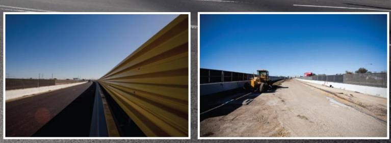
or creating temporary pavements, and having long lead in and acceleration the bridge. Bridge beams were placed on new bridge piers and concrete poured for the deck of the new bridge. Permanent 'ramp metering' traffic lights were installed on the ramps to control the flow of traffic onto the freeway. The installation of urban-art styled noisewalls made of corrugated iron and painted two different shades of yellow, will also create a new look and feel to the road.
