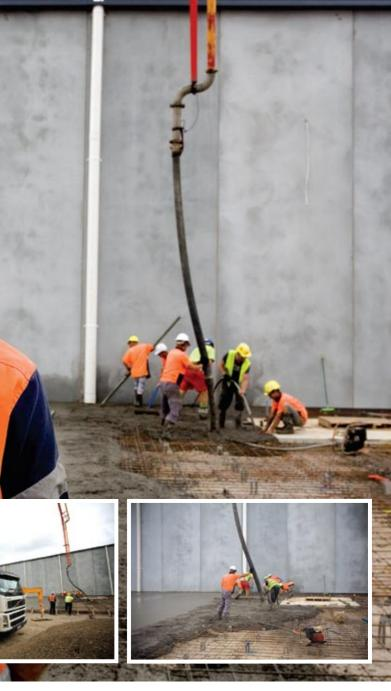
It was a large job and ACPLV used elephantine, truck-mounted 55 metre concrete boom pumps (some of Australia's heftiest) to complete it. Standard concrete placing booms ranging from 42 - 32 metre booms were also used. The job took around two months with three or four people on hand each time there was a pour.
