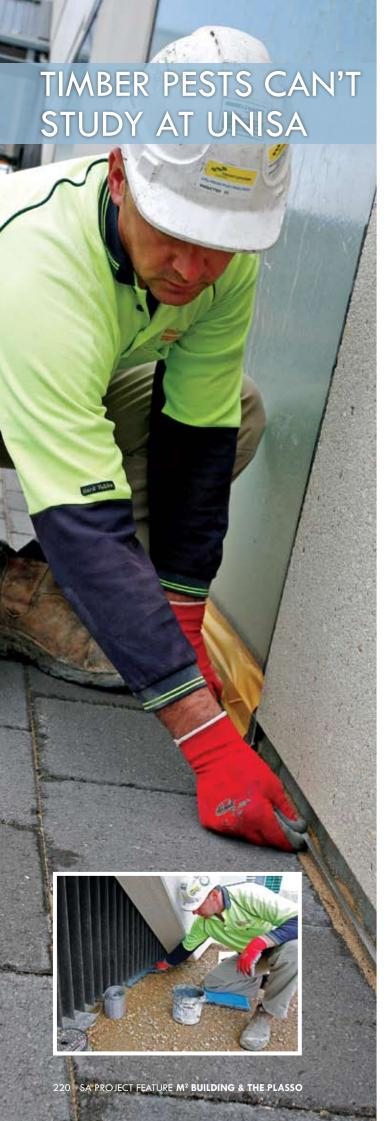
Termites are not welcome to enrol at the Uni of SA's Mawson Lakes campus, and Termimesh ensures they get turned away if the try and enter the new M² building or structures on The Plasso. Since August 2010, Termimesh's installation team have been working onsite, protecting all service penetrations within the new structure, in excess of 200m of construction joints and up to 270m of external perimeter with the company's patented stainless steel mesh barrier system.
