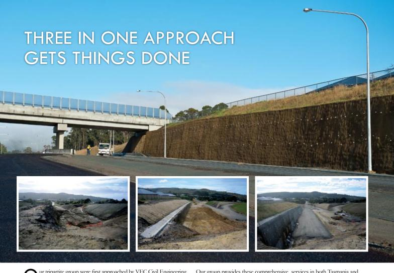
ur tripartite group were first approached by VEC Civil Engineering to submit a package to drill, supply, install and stress 7000mtrs of soil nails for the retain the shotcrete walls beneath the Summerleas Rd abutments on the Kingston By Pass project.
