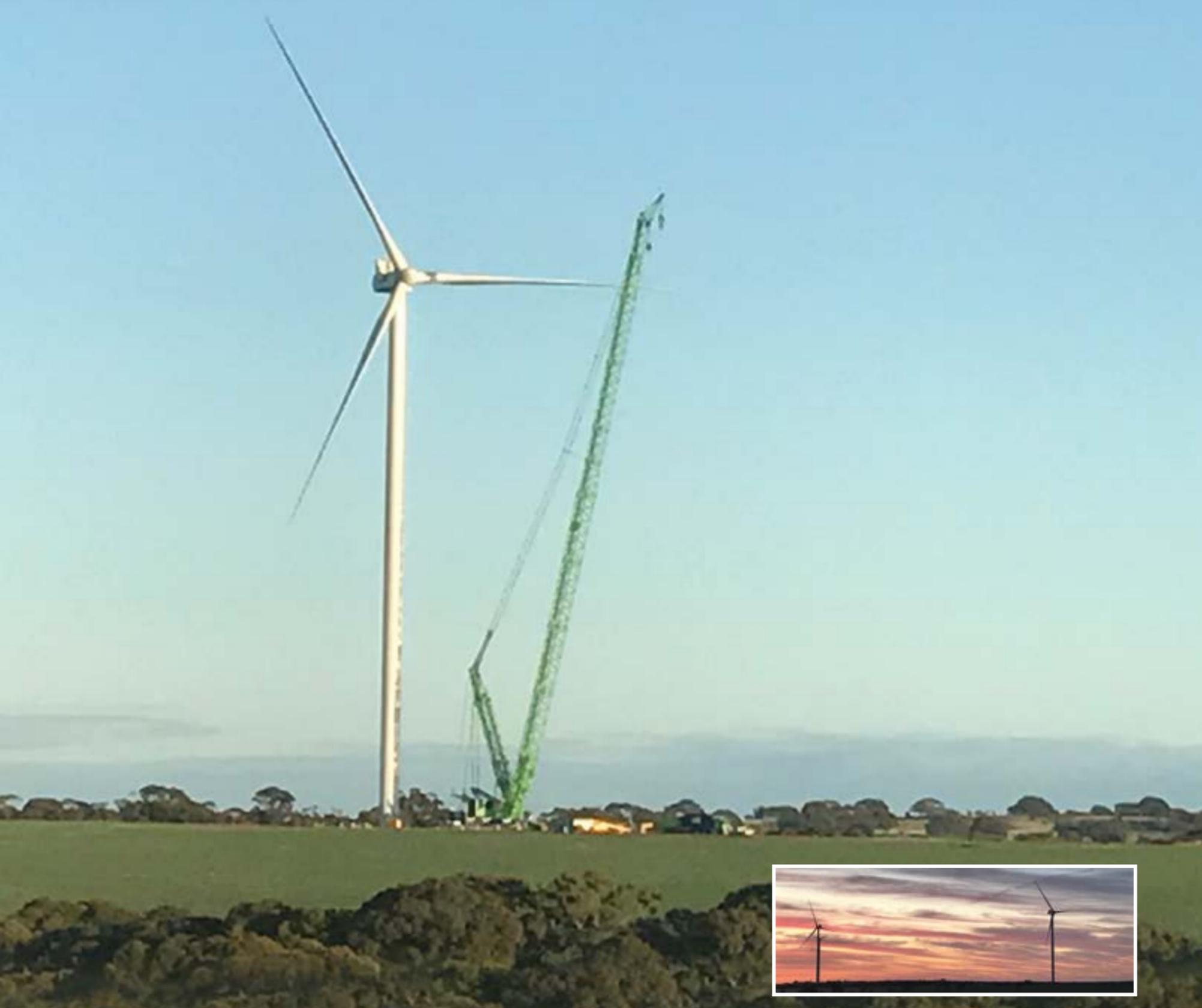
The Kiata Wind Farm consists of nine 3.45MW V126 wind turbine generators connected into the National Electricity Market through the 66KV network running between Horsham and Nhill. The project will supply enough electricity to power over 20,000 Victorian homes and will have the largest and most efficient wind turbines in Australia each standing approximately 180m tall.
