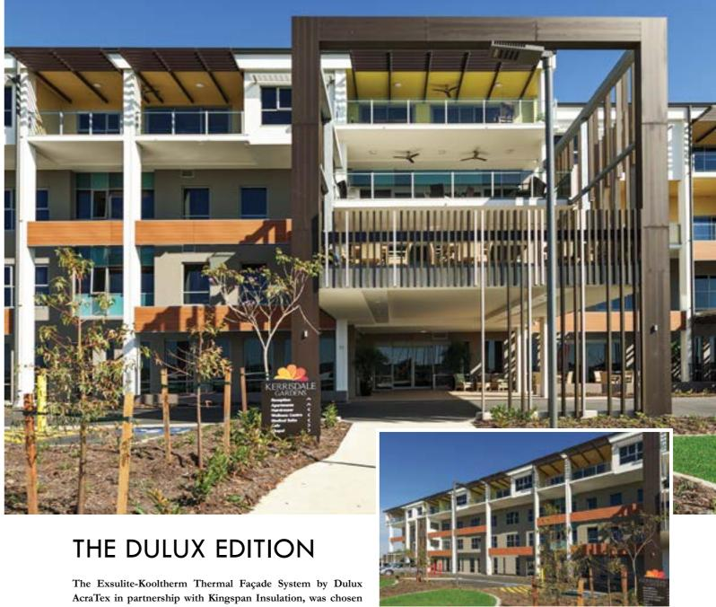
as the preferred cladding system for the Kerrisdale Gardens project. The contemporary styled total integrated thermal façade system comprises of breathable wall wrap, phenolic panels, fixings and weatherproof coatings which help to reduce maintenance and withstand the harsh climatic environmental conditions it is exposed to.
