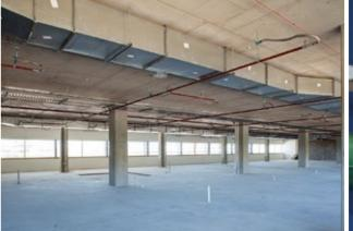
For a university located in the tropical environment of Townsville, keeping both indoor temperatures and also energy consumption down is vital, which is why RST Air Conditioning delivered a unique design for the JCU Clinical Practice Building, which uses the university's existing chilled water ring main to cool the air.
