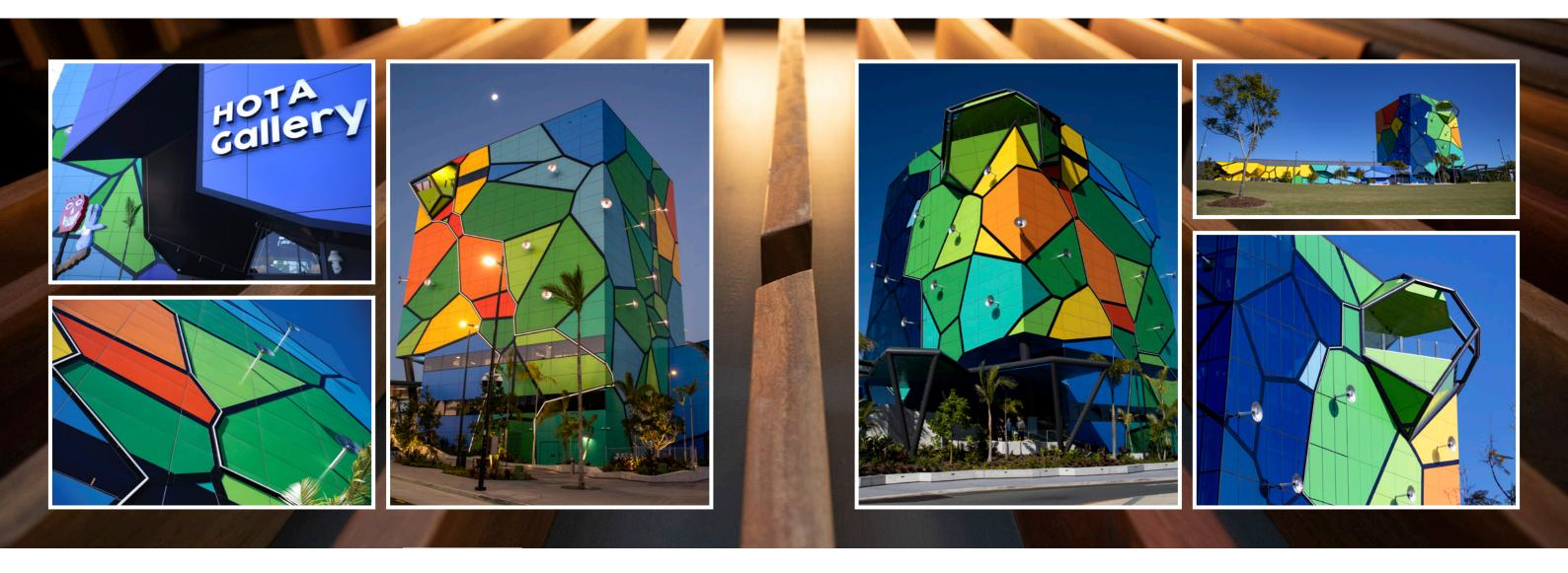
The stunning façade of the HOTA Gallery in Surfers Paradise has been constructed using high grade, fire safe SAP aluminium panels supplied by locally based Aodeli Australia, a leading supplier of aluminium architectural cladding solutions which meet Australian Standard AS1530.1 for non-combustibility.
