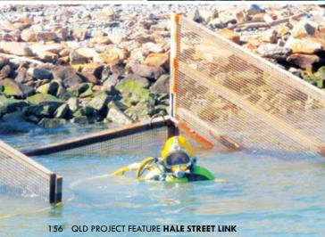
orking underwater in the dimness of the Brisbane River, Dermody Diving and Marine Services (DDMS) undertook essential diving support work for the Hale Street Link project including inspections, welding, cutting and lifting operations, Pile protection and wrapping system.
