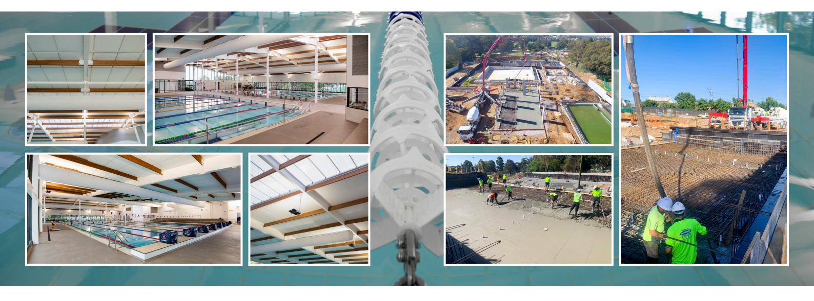
The Goulburn Aquatic and Leisure Centre boasts a host of new facilities including a new eight lane indoor pool, warm water pool, change rooms and associated facilities. The roof structure of the main pool hall is comprised of a primary steel structure with glue laminated timber (GLT) purlins which were provided by mass timber manufacturer XLam (xlam.com.au). The use of timber created an elegant architectural statement, introducing warm, natural tones into the project.
