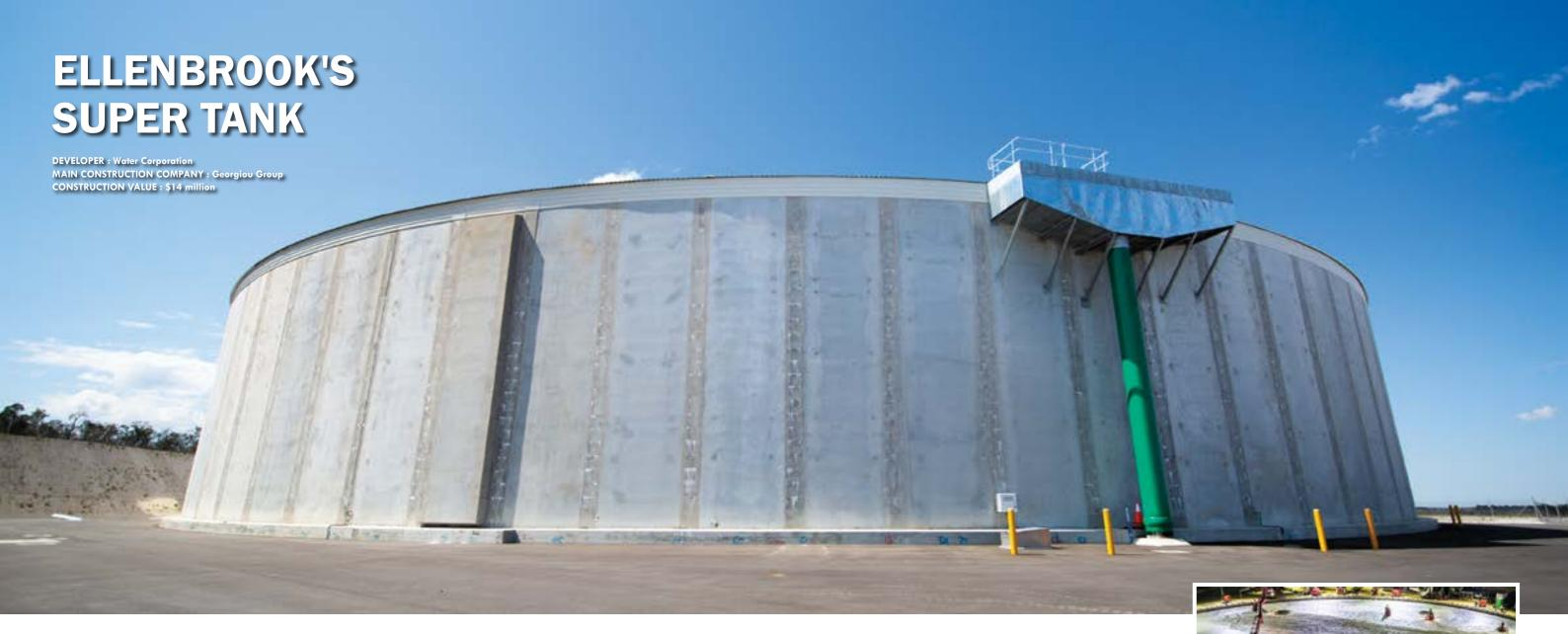
The 80 million litre Ellenbrook Tank, contains enough water to support the growth of Ellenbrook and the north eastern metropolitan corridor. Measuring approximately 90m in diameter and 14m in height it is the largest concrete tank Georgiou Group and the Water Corporation have ever constructed.
