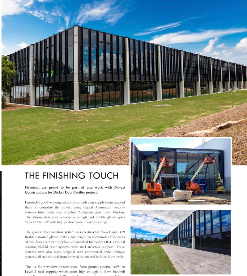
compliance on the roof. The window system is constructed from the Capral CW150 Curtain Wall System. The system consists of vertical heavy duty captive window mullions integrated with non-captive horizontal transoms. The system has been engineered and had a custom designed vertical feature fin added to conceal all support fixings externally.
