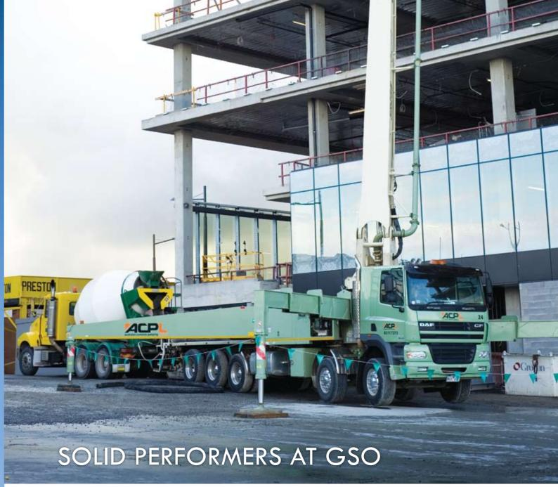
To ensure efficient and safe placement of the concrete for the Dandenong GSO project, Grocon relied on Australian Concrete Pumping Logistics (Victoria) to provide mobile boom concrete pumping plant and equipment on a daily hire basis.
