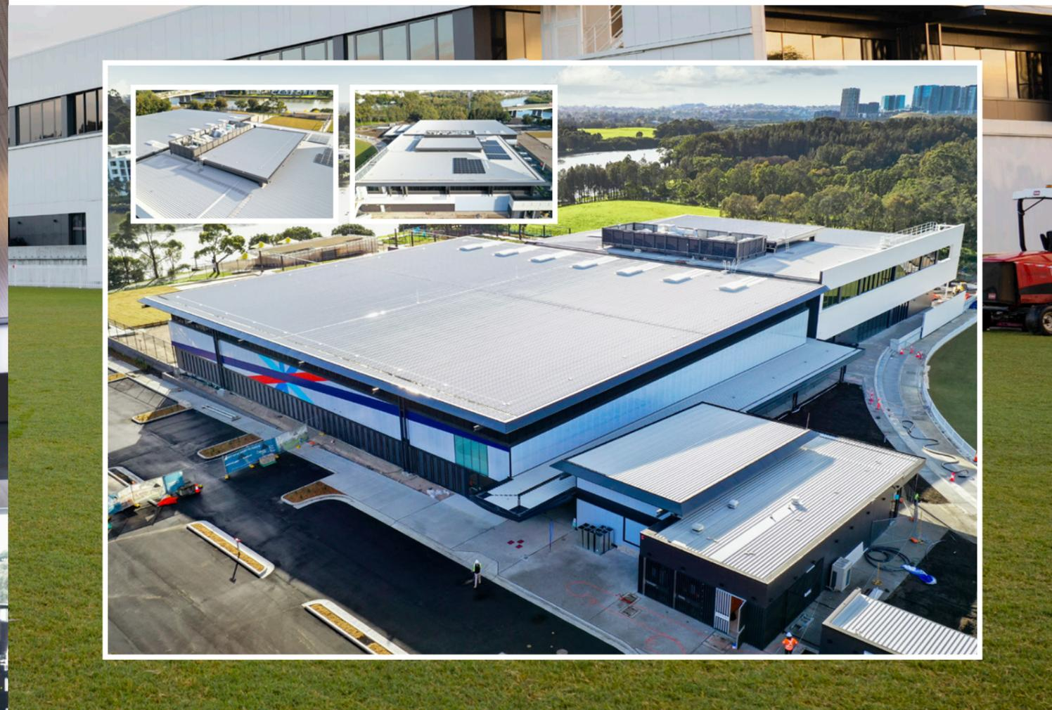
Cre8tive Roofing Services was contracted to deliver all of the roofworks, box gutters, flashing and Danpalon cladding for Cricket Central.
