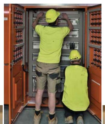
Pope manufactured a pressurisation control system with four pressurisation fans which controlled the central pressure of the stairwell, as well as regulating two smoke spill exhaust fans. "The system used ABB variable speed drives, the Eliwell system and four Dwyer static pressure transducers," Bradley said.
