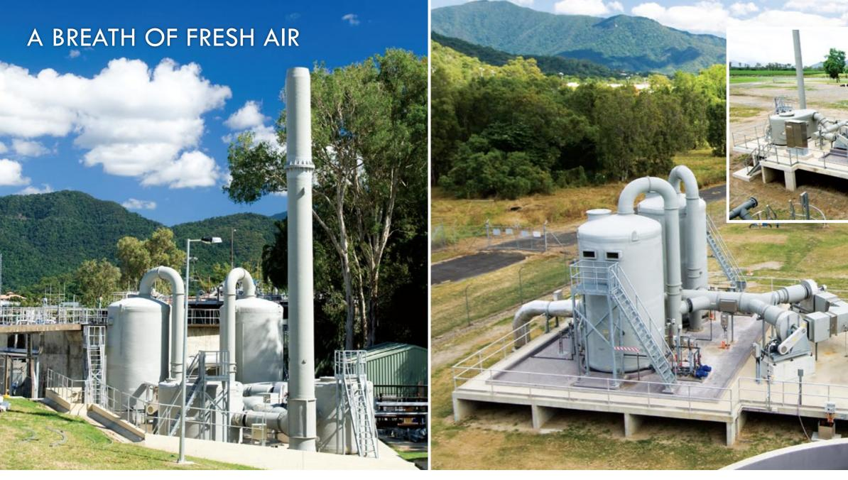
aste Water Treatment Plants can get awfully whiffy; fortunately, when the balmy tropical breeze blows around Cairns, technology by Aromatrix ensures there's no unpleasant odours from the newly upgraded Marlin Coast, Northern or Southern WWTPs. Aromatrix engineer leading edge odour control technologies based on bacterial action and activated carbon, rather than harsh chemicals. This approach makes their process an ecologically safe choice for the adjoining Great Barrier Reef Marine Park.
