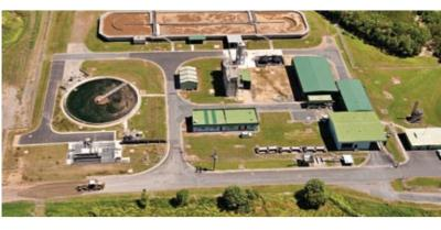
This process, commonly referred to as "MBR", uses ultra-filtration membranes to provide high-quality water that meets Queensland Class A recycled water standard (after chlorination)," said Sam.
