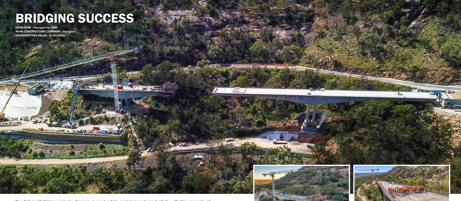
The Bolivia Hill Bridge project will improve road safety and transport productivity with the upgrade of 2.2km of the New England Highway and the construction of a bridge approximately 320m long. Including the widening and realigning the existing two-lane highway, and the regrading of temporary access tracks to provide permanent 4WD drive access, the project will improve road safety and road transport productivity.
