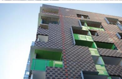
Turning innovative architectural designs into precast concrete achievements is what Westkon excel at. Their ability to deliver extremely complex structural solutions is showcased beautifully in the Atherton Gardens project, where they provided concrete elements for the façade and internal lift shafts.
