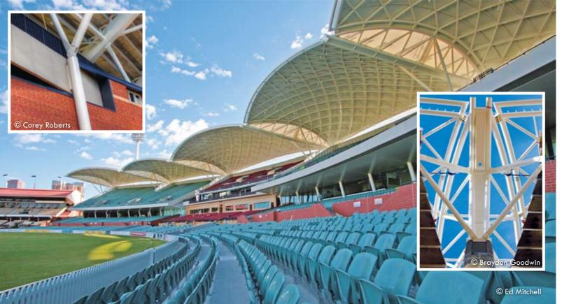
"We decided the most appropriate response was to break down the scale of the facility from what could have been one single element (so common in many contemporary stadia designs due to efficiency), into five separate bays, with a larger "pavilion" in the centre flanked by two smaller bays either side. The resulting scale of the smaller pieces is more suited to the smaller series of buildings and stands present on the site.
