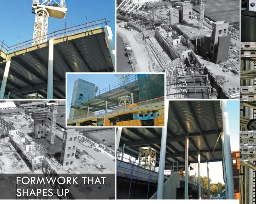
hen concrete's ready to pour, the formwork's got to be ready to hold it, and on a major project like the Adelaide Oval's Western Grandstand, that takes the combination of skill and logistics Newgen Formwork bring to a site. Newgen supplied and installed all the suspended formwork for the Western Grandstand, suspended stairs, two 30 metre lift cores and all the concourse seating plats.
