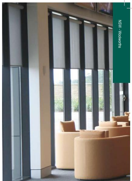
stallation of five 14m high motorized roller blinds for the entry area. This involved reconfiguring the drive motors to ensure there was adequate torque and reliability as well as working at a considerable hight, which required intensive OH&S documentation and planning.
