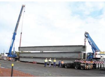
Top 2 x 20 tonne Franna cranes loading barge with water piping for installation under Tourle Street Bridge
