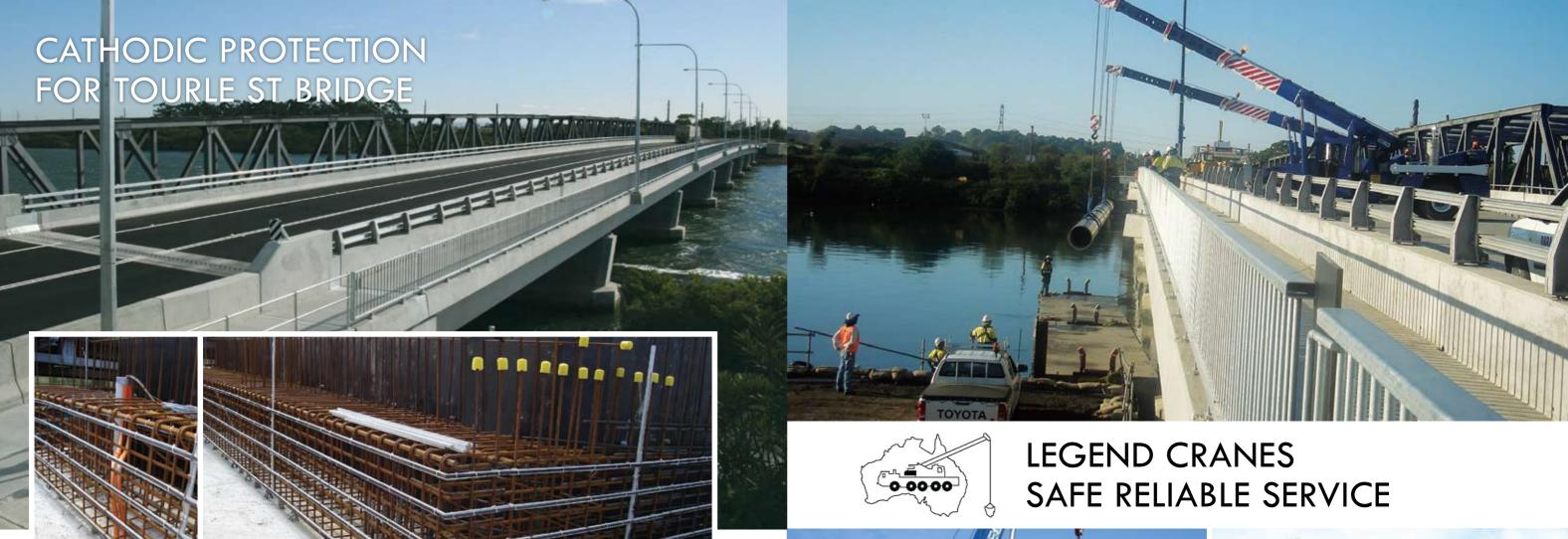
orrosion Control Engineering (NSW) Pty Ltd were engaged by ■ Daracon Contractors in December 2008 to re-design, supply, install and commission an Impressed Current Cathodic Protection (ICCP) System to the new Tourle St Bridge, which runs over the Hunter River in Mayfield, Newcastle.
