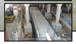
to get the shutters for the formwork in place, due to the limited height, which was only 4 metres of height inside the building, but there was a 7-metre trench to dig. Access was the biggest problem, as all the work had to take place inside the building, while the plant was still operational.
