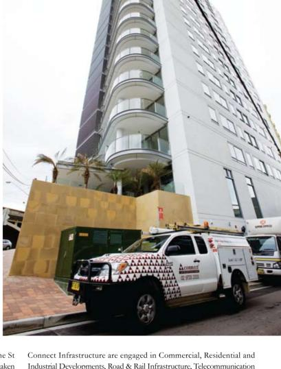
The installation of the 800kVA kiosk substation as part of the St Hilliers refurbishment of 118 Alfred St Milsons Point was undertaken in concept, design and construction by Connect Infrastructure.
