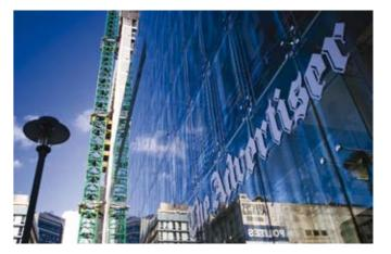
two layers of glass in the façade is a 1-metre wide walkway to enable cleaning.
