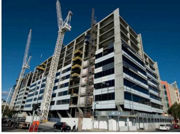
Another challenge facing the company was the construction of the massive Y shaped concrete columns on the Precinct C project. The unique Y column structural solution, used instead of a traditional ground level slab, is designed to take the loads from the upper floors and distribute them into a single point at the base of the Y, simplifying the transfer of the structural load down to the foundations and creating a less cluttered look at ground level.
