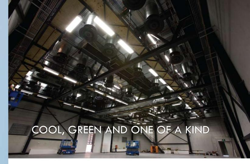
A ustral Air Conditioning Services supplied and installed a world first cooling system for Global Television and Channel 7 Studios at 8 Central Avenue, Everleigh. The system had to be very quiet and able to cool extremely high temperatures created by studio production lighting.
