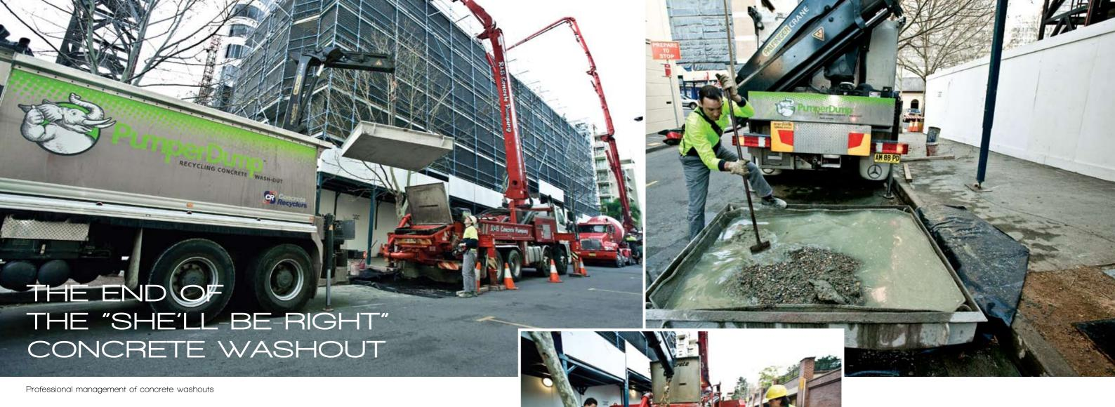
oncrete pour washouts on Lipman's major King Street, Sydney CBD project were faster and more efficient thanks to the unique PumperDump system. Usually, such Group A waste run-off (pH >12–14) from site wash-down areas poses both an environmental and logistical challenge.
