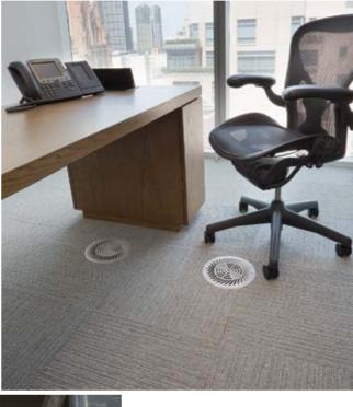
air leakage performance achieved on site is 0.3-0.4L/second/m<sup>2</sup>, which is extremely low and adds to the energy efficiency of the UFAD system.
