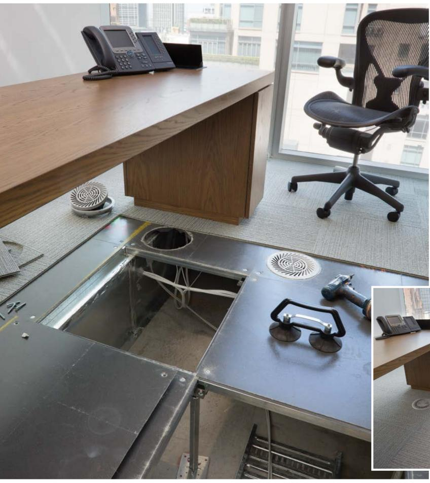
When technology changes, as it inevitably will, the proprietary flooring system installed by Tate Tasman Access Floors (TTAF) at 171 Collins Street means occupants can move with the times, without having to dismantle sections of the walls or ceiling to do it.
