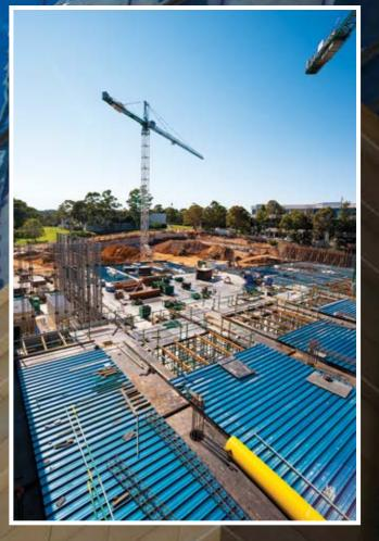
De Martin and Gasparini (DMG) were awarded the contract for all in-situ concrete works required for the 161 Castlereagh Street, Sydney project. The scope included the supply, pump, place and finish of approximately 36,000m³ of concrete. The project brief required the supply and delivery of high strength, high performance 'green' concrete, having no less than 20% cement and 20% aggregate replacement, without compromising structural integrity.
