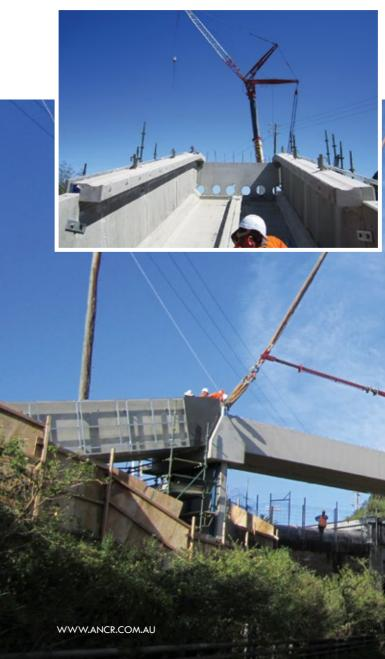
concrete units. Westkon worked in consultation on the development of the design, in particular, regarding the detail of the shear reinforcement in the beams. This challenge concerned the removal of any chance of the beams themselves becoming transformers for the electrical conduit, which may have occurred had any of the pre-stressed reinforcing had any closed loops.
