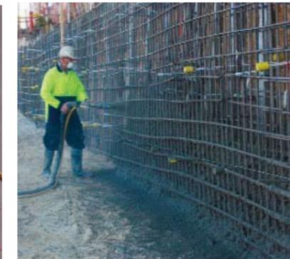
**ABOVE:** PREPARED RETAINING WALL BEING SPRAYED LEURA BY PASS.
