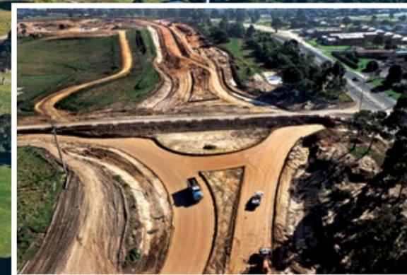
BMD's Princes Highway East Duplication – Wurruk to Sale section comprises 4.5km of dual carriageway, four new road bridges, 6 refurbished road bridges and an architecturally-designed 90 metre cable stay pedestrian bridge.
