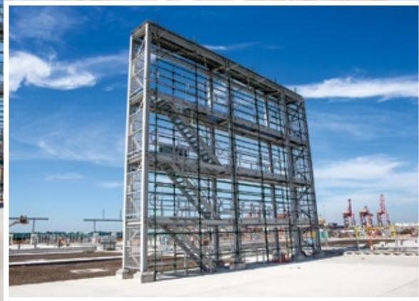
Decades of solid experience in meeting the needs of projects with stringent standards makes NWEC a preferred structural steel subcontractor for projects like Port Botany T3, where their scope included fabricated and installing 160T of structural steel for the substations, Reefer Gantries and Walkways. All items were surface treated with either three coat epoxy or galvanised due to the corrosive coastal location, giving the painted structures a design life of 100 years.
