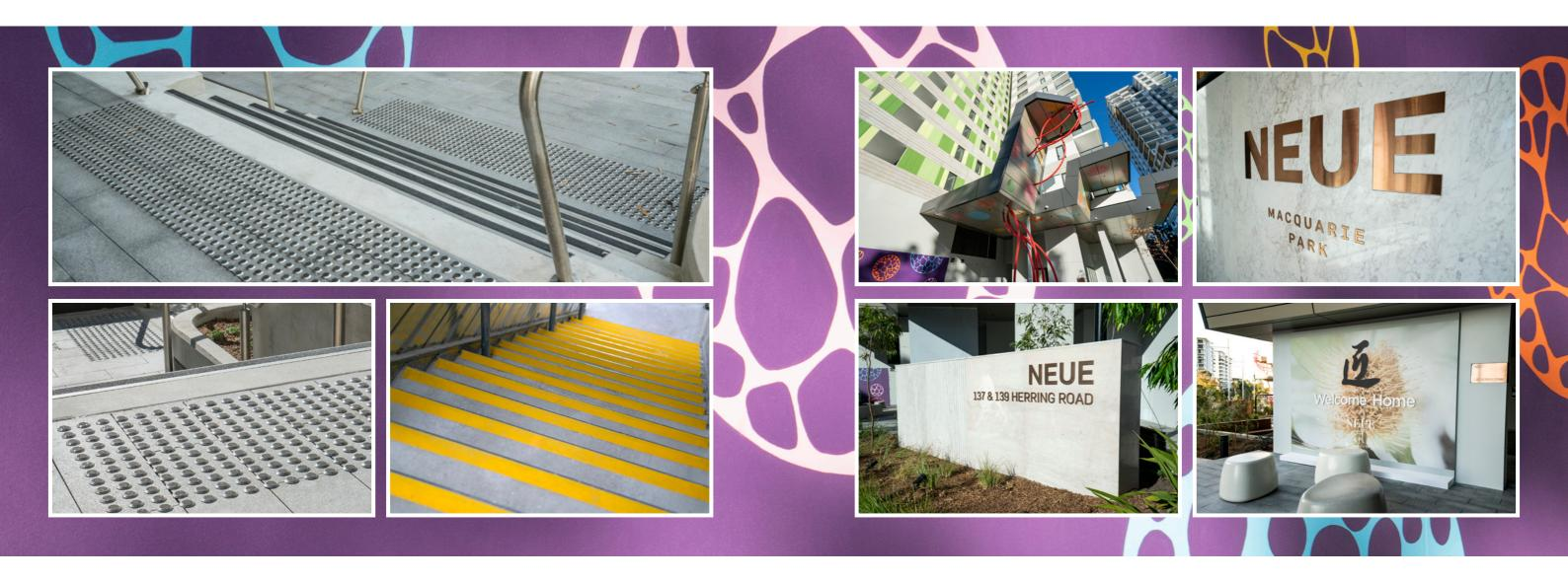
The mission of Safespot Architectural Products is to facilitate safe and independent access to the built environment for blind and vision impaired people through the supply and installation of Tactile Ground Surface Indicators (TGSIs) and stair nosings.
