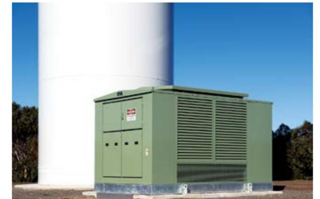
2.6MVA 33kV/690V kiosk transformers with HV switchgear for Meridian Energy's Westwind Wind Farm in Wellington New Zealand, 9 No. 1.0MVA 33kV/690V Kiosk Transformers with HV Switchgear to Pioneer Generation's Mt Stuart Wind farm in Otago, 55 No. 800kVA 33kV/690V Kiosk Transformers with HV Switchgear to Trustpower's Taurua Wind farm on the Taurua Ranges and 5 No. 2.5MVA 33kV/690V DSTATCOM HV/LV cablebox style transformers for AGL's Oakland's Hill wind farm substation in Victoria
